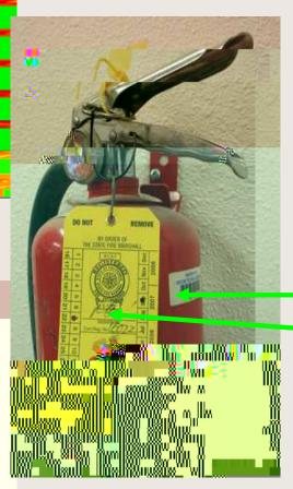
The nozzle should be clear of blockages. Signs of yellow powder could also indicate a leak or tampering and should be reported.
